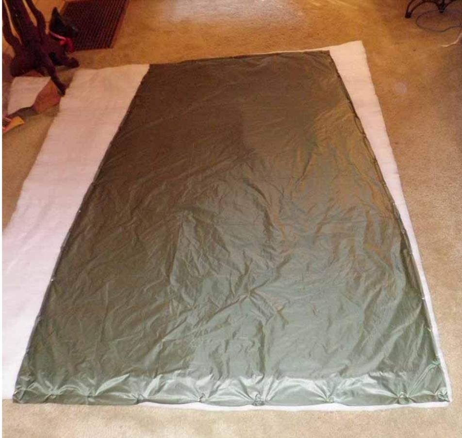
Figure 3 Pin the panels on top of the insulation.
